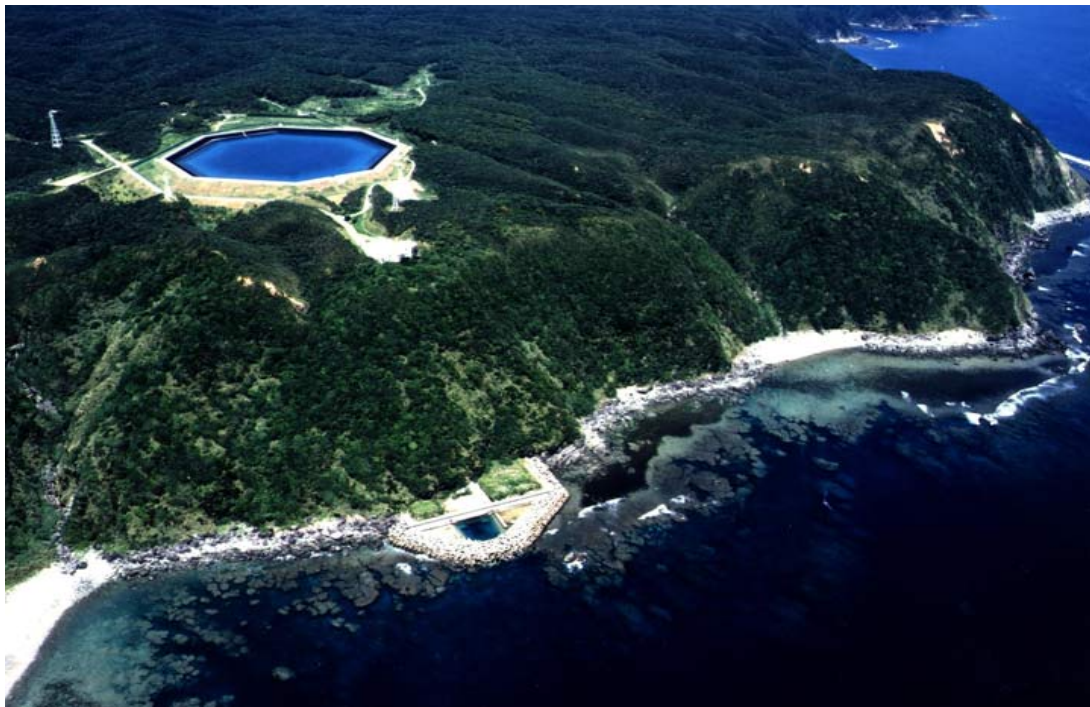
In this pumped storage system in Okinawa, Japan, seawater is pumped up into a single reservoir, and released again when energy is needed.
